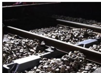
The installation of the test track in Kalmar was done overnight on the 28th of April 2016. The section is already successfully in service. Lankhorst's KLP® Hybrid polymer Sleeper and 5 other alternative sleepers were installed by Trafikverket.
