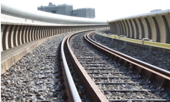
KLP® Hybrid Polymer Sleepers installed in Amsterdam (light rail)
